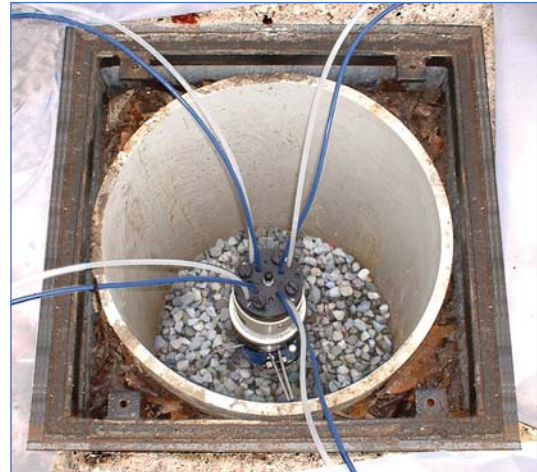
Multi-Purge Manifold with Transducers and Dedicated Pumps for four zone monitoring
