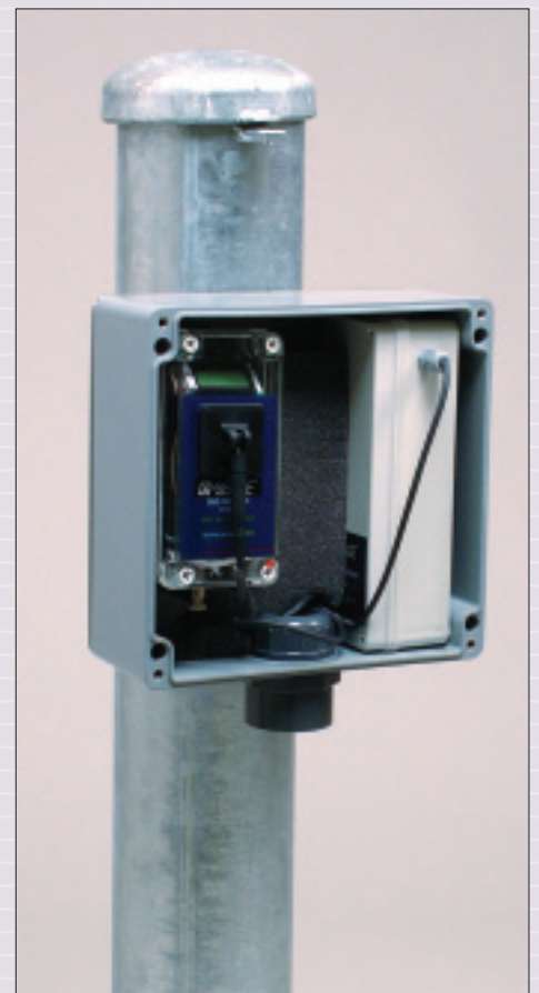
Above-ground housing connected to a monitoring well cover
