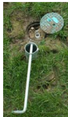
Fig. 4 One central ground anchor installed under the engine
