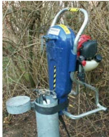
Fig. 3 Strap fixed around casing
