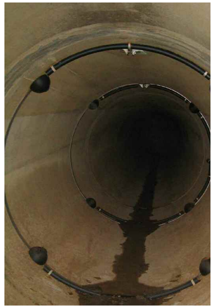
Pressured pipe, Evora
