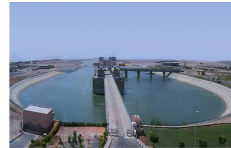
Mubarak Pumping Station, Egypt
